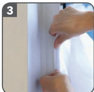
First stick the wide **side A** (zipper is closed) with open windows from the middle to the left and right side or to the up and down side to the window frame.
